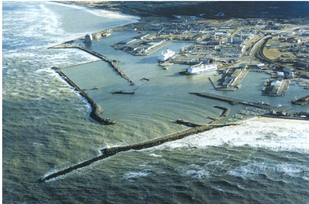
Hirtshals Harbour: Breakwater
