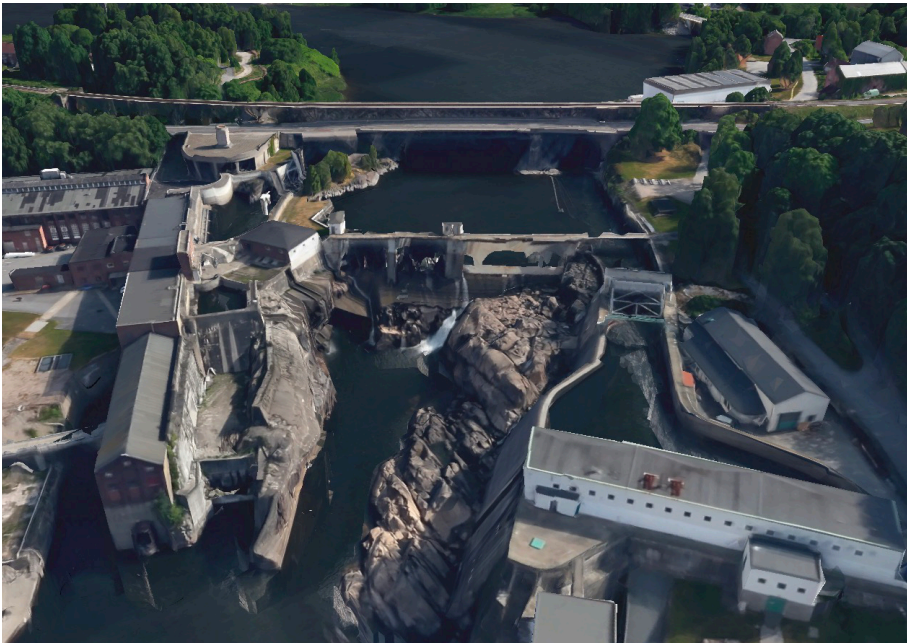
Sarpfossen Hydropower Plant
