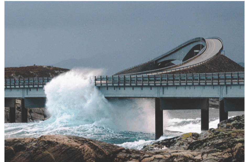
Coastal Transportation Infrastructure
